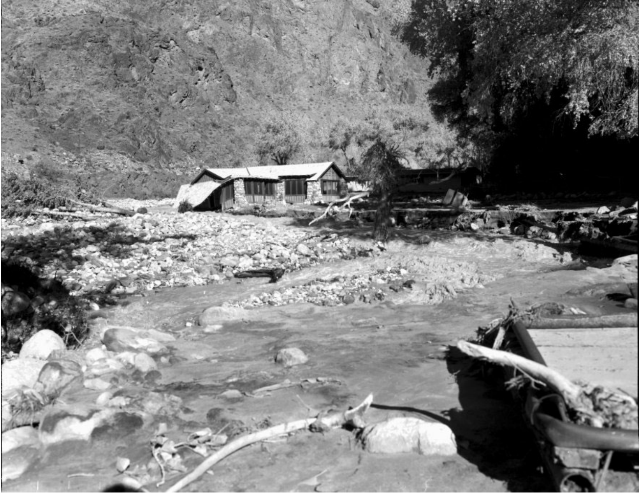
#5099:...and damaged the NPS Bunkhouse building.
