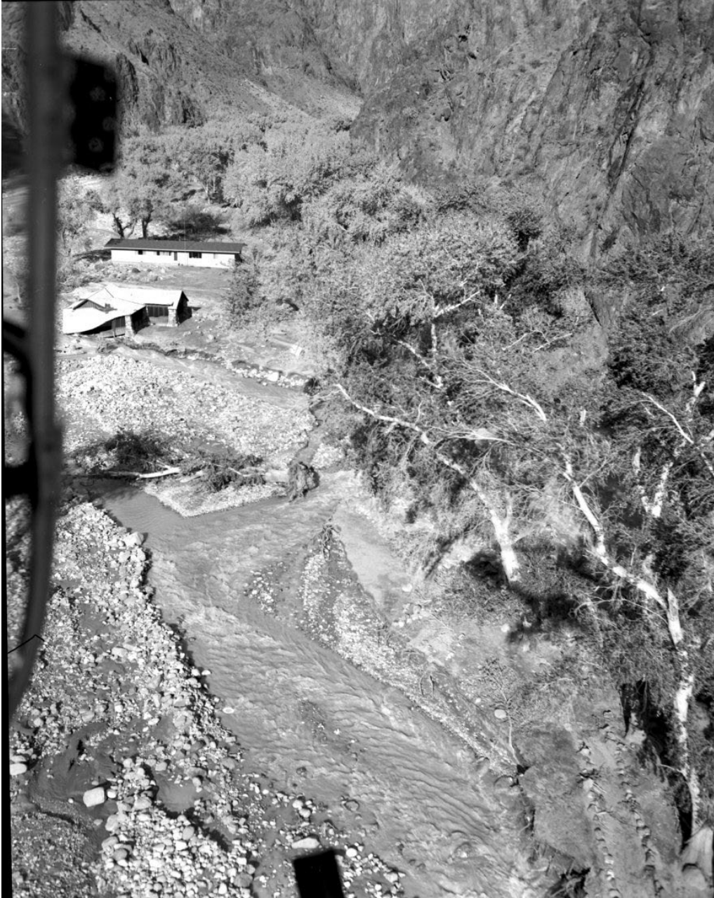
#5098 Flash flooding in the spring of 1966, caused Bright Angel Creek to change its course...
