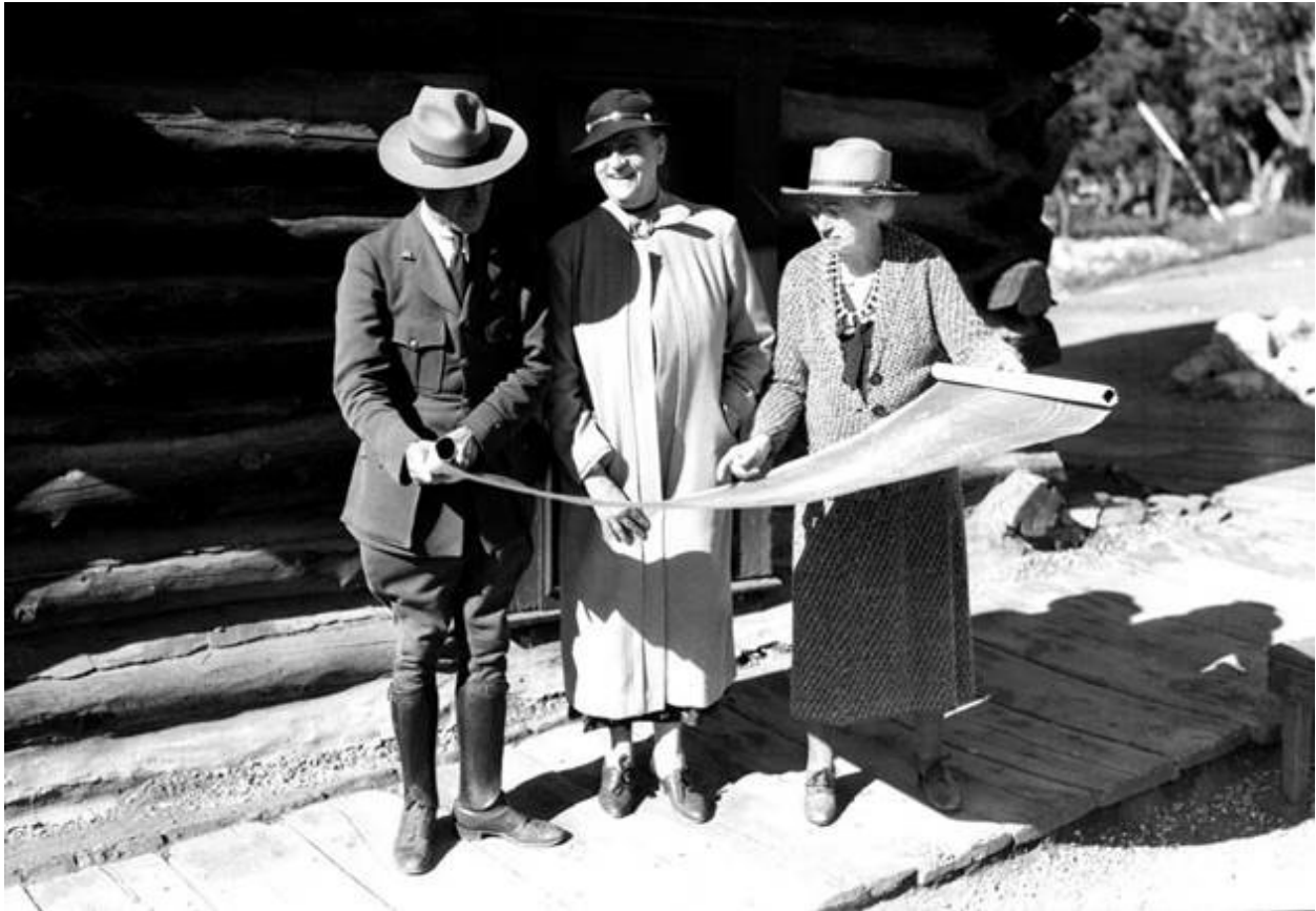
#16942: SUPERINTENDENT TILLOTSON, MRS ICKES, & MARY COLTER LOOKING AT CONSTRUCTION PLANS, CIRCA 1932.
