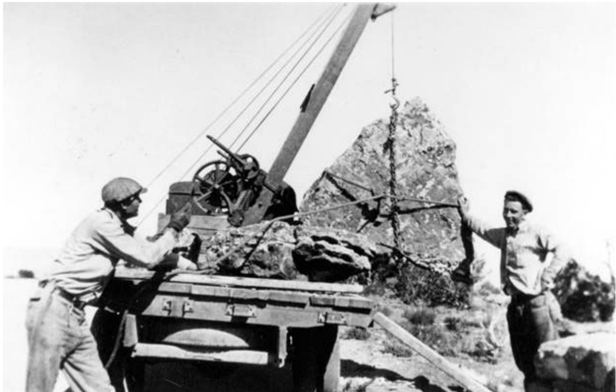
#16978: MEN USING WINCH TO PUT ROCKS IN PLACE DURING WATCHTOWER CONSTRUCTION, CIRCA 1932.
