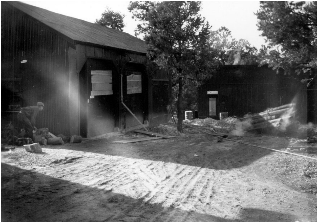
#00302: BLASTING ROCK TO LAY WATERLINE TO NEW DARKROOM, CIRCA 1932
