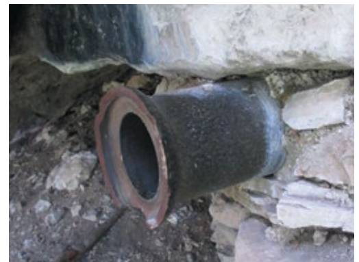
Fig. 3. The two sidewalls used to convert the cliff overhang into a “shelter” each include a ventilation pipe having an inner diameter 14 cm. The pipes project 0.3 meters from the shelter’s walls. (Photo by Randy Moore)
