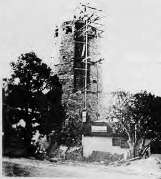
Watchtower at Desert View under construction.
