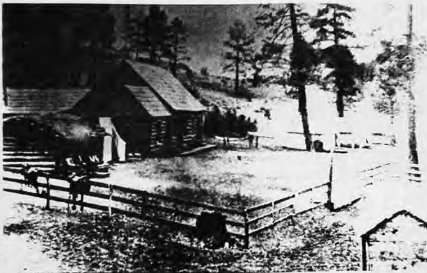
The Hance Cabin as it appeared around 1885.
