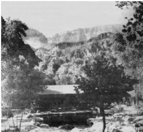
The swimming pool and the recreation hall at Phantom Ranch, Grand Canyon as it appeared January 22, 1965
