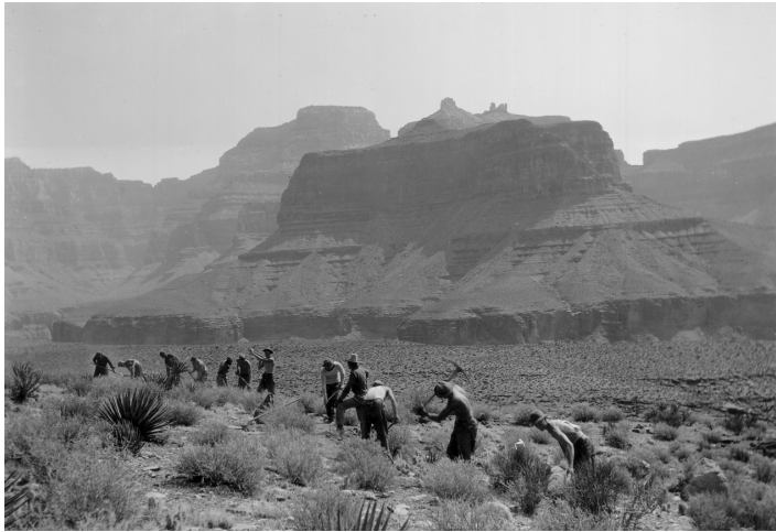
CCC Workers on the Clear Creek Trail
