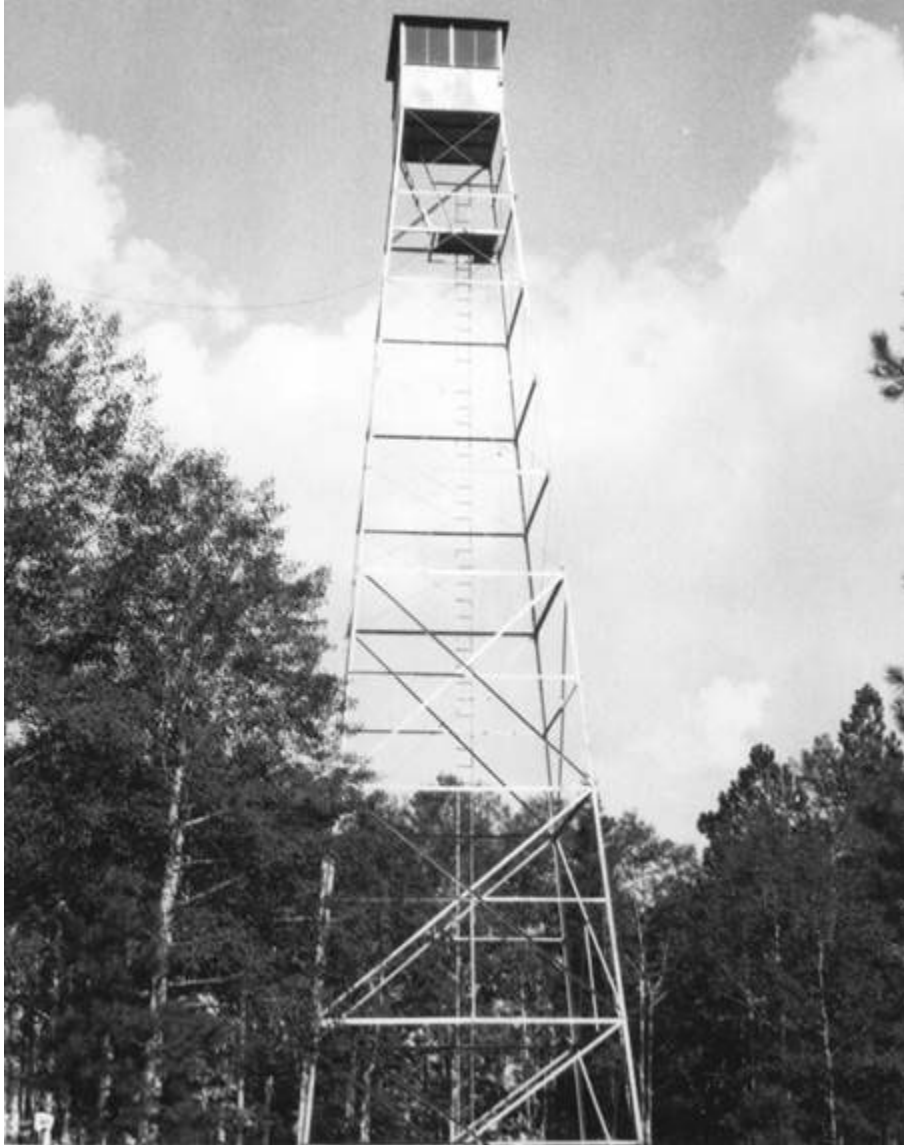
#03930: BRIGHT ANGEL POINT FIRE TOWER AFTER BEING MOVED 12 MILES NORTH, CIRCA 1933
