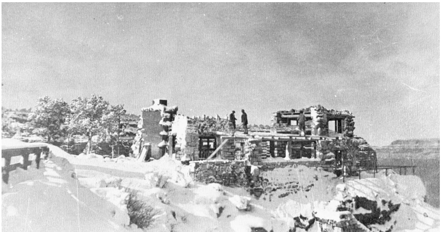
Figure 1. The Lookout under construction, c. 1914. Note the original wide brick chimney that was removed and replaced with a narrower stone chimney during construction. 13336 Grand Canyon Historic collection.
