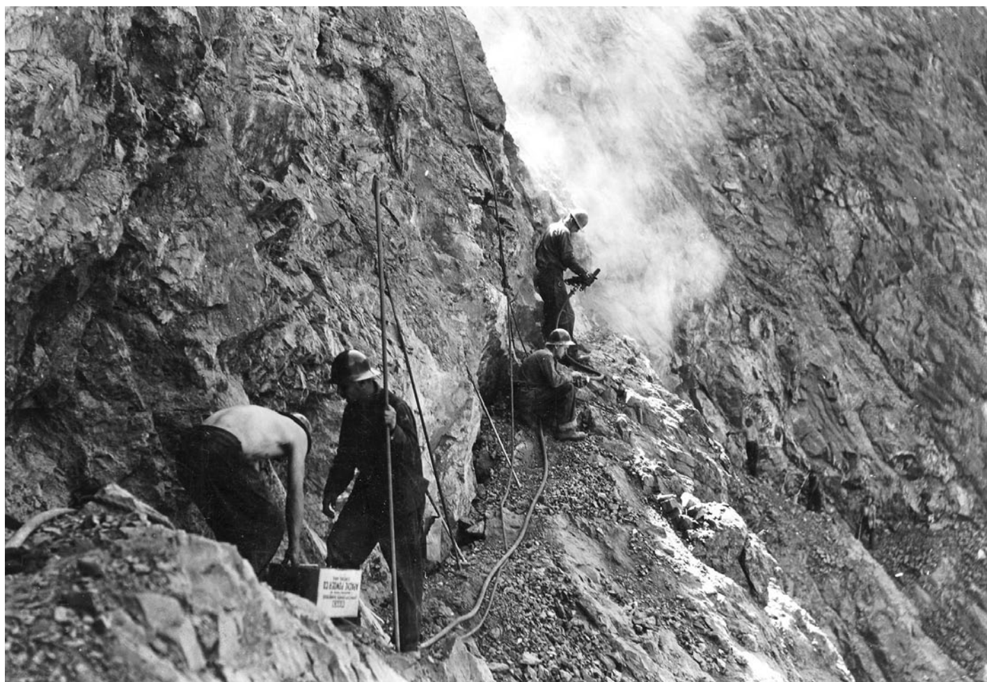
Construction of River Trail by CCC enrollees. Enrollees working on ledge. Blasting area. Circa 1935. NPS.
