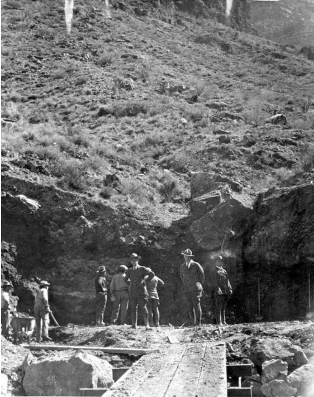
#00085: NPS OFFICIALS AT CONSTRUCTION SITE FOR INDIAN GARDEN WATER PIPELINE, CIRCA 1932.
