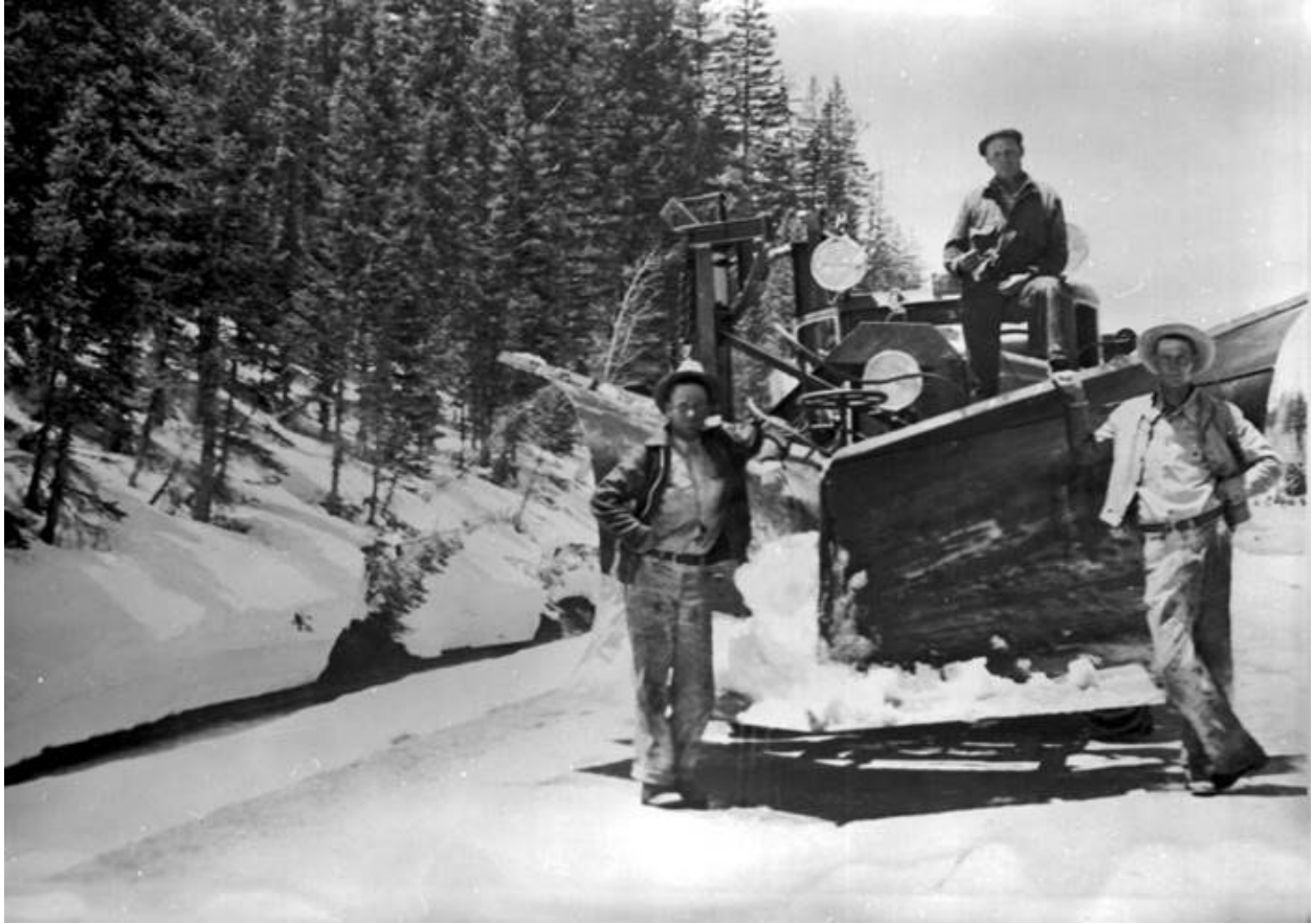
#15541: SPRING OPENING OF NORTH RIM ROAD USING A STATE HIGHWAY PLOW, CIRCA 1934. PHOTO BY WARREN HAMILTON.
