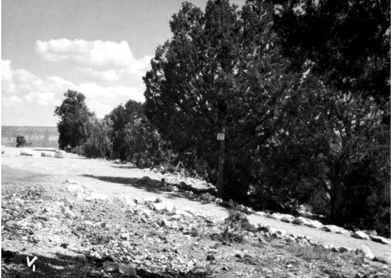
#07395: WORK ON THE FOOTPATH NEAR POWELL MEMORIAL, SOUTH RIM, CIRCA 1930
