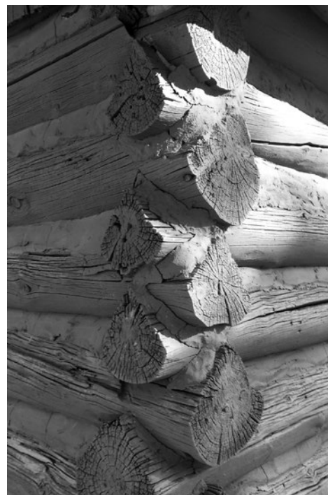
Hull (and Hance) Cabin saddle notching
