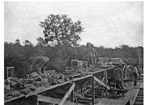
Figure 8 - Masons Laying Stone at Hopi House - 1904 - Mennonite Library and Archives, Bethel College, North Newton, Kansas.
