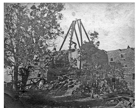
Figure 9 - Wooden Gantry Crane at Hopi House - 1904 - Mennonite Library and Archives, Bethel College, North Newton, Kansas.
